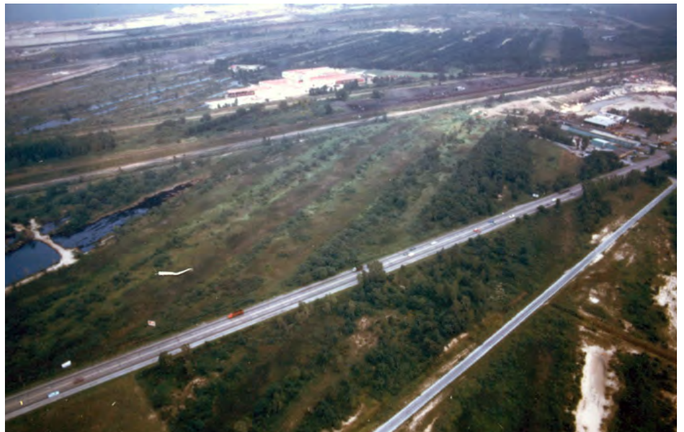
Poorly-sited infrastructure is a common driver of landscape fragmentation, as with these parallel highways at the Indiana Dunes National Lakeshore in the USA.
