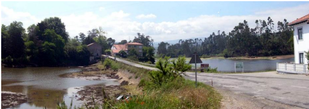
Fig. 70. Road barrier effects are varied. Road embankments affect tide cycles and therefore inland wetlands biodiversity in this estuary of La Rabia, Cantabria (Spain). (Photo by I. Español)
