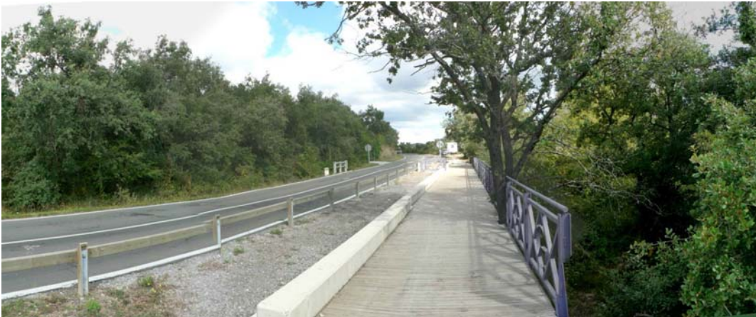
Fig. 50. Separate bicycle lane. Safety barrier and low parapet separate pedestrians from traffic. (Photo by I. Español)
