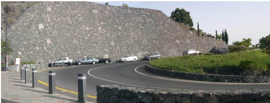
Fig 63. Parapet in the foreground is a traditional stone wall together with modern materials like prevention posts. In the background a retaining wall is covered with a traditional black stone wall, while at margins gardening includes local plants and big rocks as well. All these elements together manage to create a sense of road identity. (Photo by I. Español).
