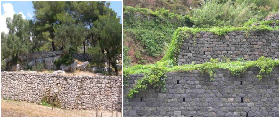
Fig. 22 and 23. Traditional stone walls are features of landscape character. (Left) Walls made of dry limestone are a traditional feature of Ise of Mjlet (Croatia). (Right) Characteristic retaining walls made of volcanic stone for vertical vineyard embankments on the island of Madeira (Portugal). (Photos by I. Español)
