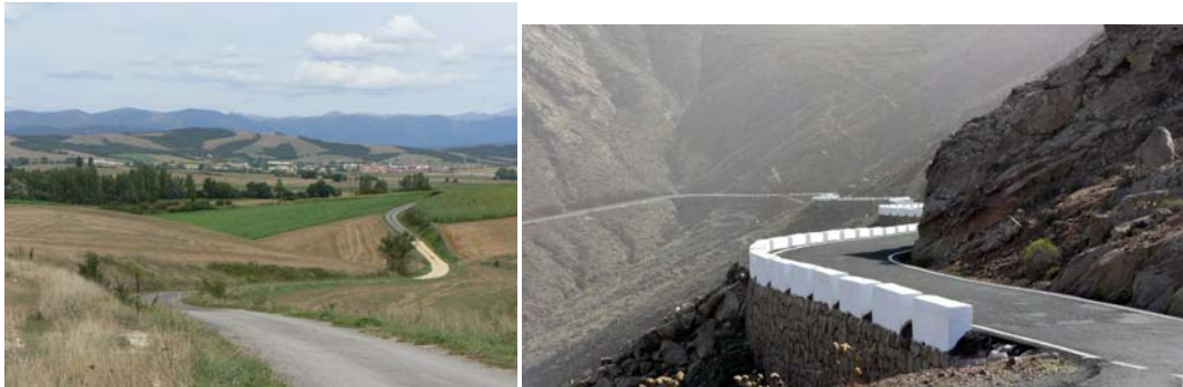
Fig. 74 and 75. The linear effect of a road can emphasise landscape composition by giving a sense of depth. (Left) The alignment of a small road shows morphology by providing a continuous reference to the observer along the hills. (Right) Linear presence of roads, reinforced by “teeth-like” parapets, gives a sense of depth and real relief. (Photo by I. Español)
