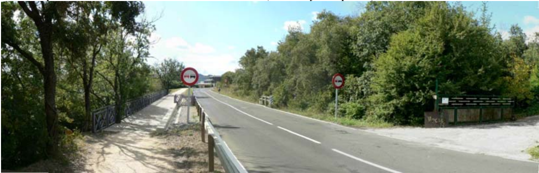
Fig. III-10. The side platform (on the left) respects vegetation on both sides of the road, encouraging ecological connectivity underneath. (Photo by I. Español)
