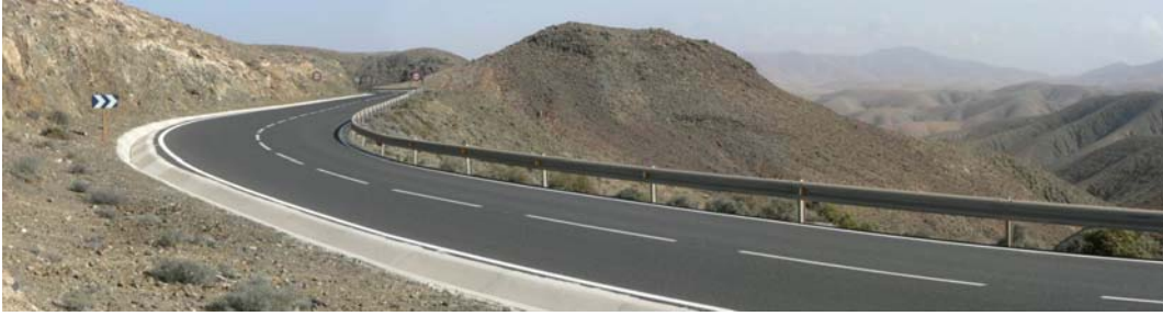
Fig. 67. The linear character of roads determines their role in landscape. Road environment effects on landscape processes, the scenic presence of roads, together with the effect of roads on landscape perception are based mainly on their linear condition. (Photo by I. Español).
