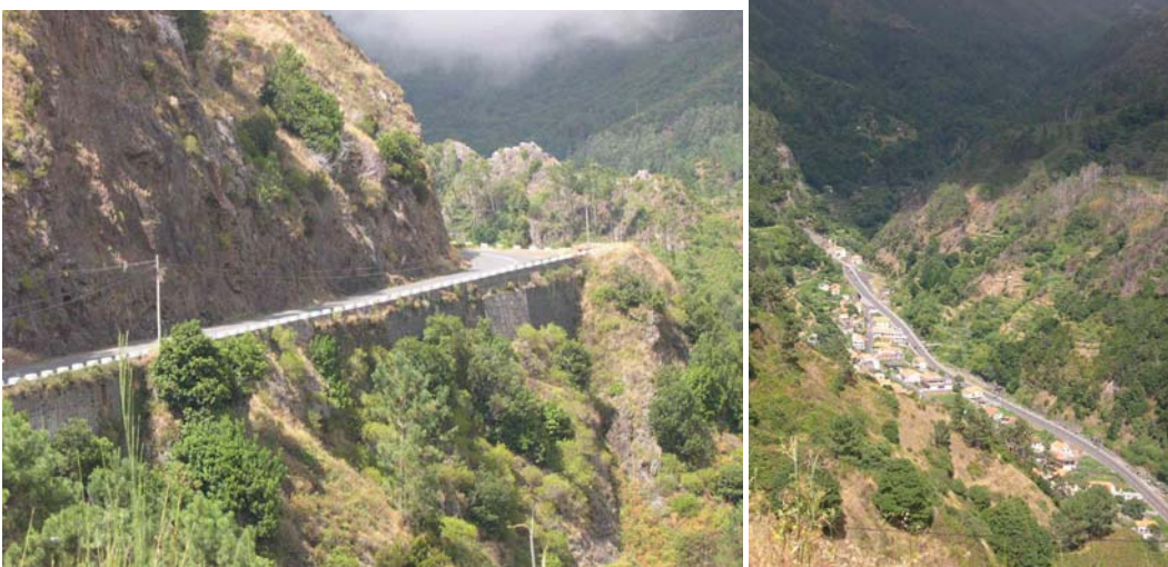
Fig. 68 and 69. Roads on the slope and at the bottom of a valley in Serra de Agua, Madeira, Portugal. (Photos by I. Español) A variety of road environmental effects should be taken into account. (Left) Short term effects: water aquifer reserves can be drained by the effect of road cutting at the base of the aquifer formation. (Right) Roads are an axis for human activity which must be taken into account by strategic planning.
