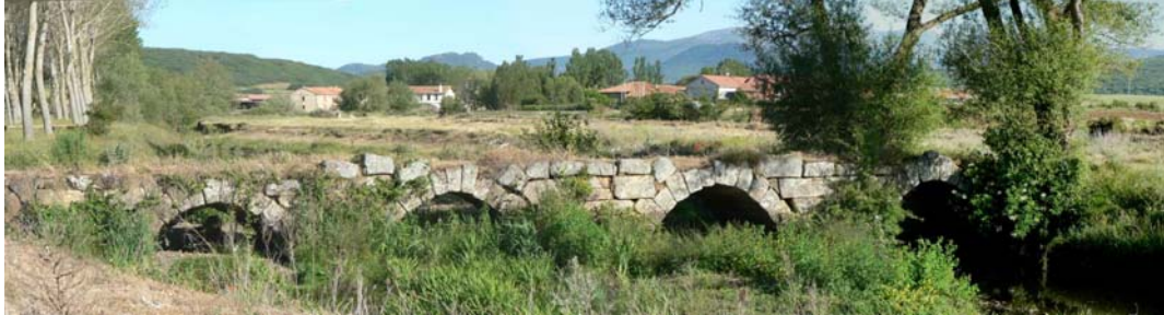
Fig. II-3. Stone bridge of Roman origin on the Rubagon River at Nestar. The Roman road to the Northeast and current P-220 road run parallel to the river to the left of this picture. The Roman road to Cantabria diverted here. (Photo by I. Español)
