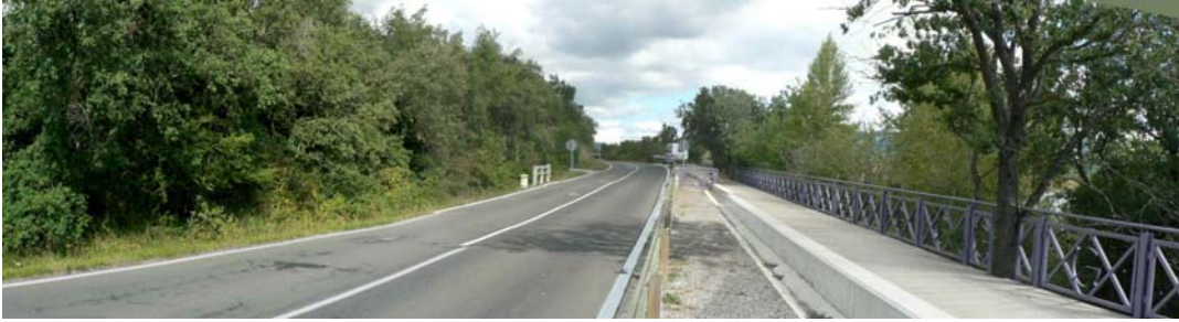
Fig. III-8. A footpath has been included along the itinerary of the A-3002 a side platform. A white parapet and a safety barrier separate pedestrians from traffic and a banister prevents access to the shore. (Photo by I. Español)
