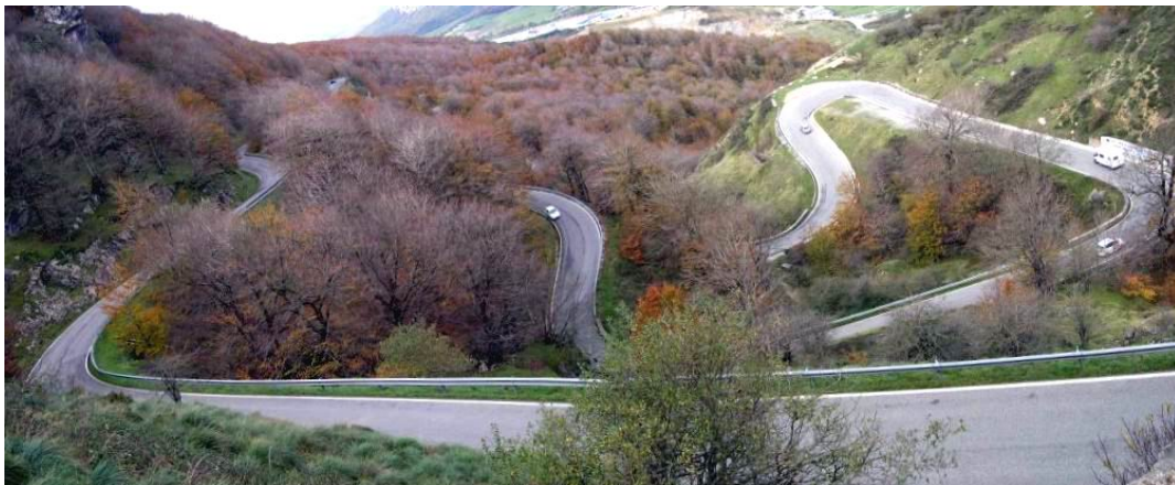
Fig. 15. Road from Altsasua to Olazagutia (Navarre, Spain) Mountain roads, curved and steep alignments prevent sightseeing, despite the impressive views available from the road. (Photo by I. Español)
