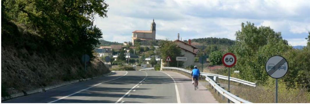
Fig. III-1. The A-3002 road in Alava (Spain) has a good scenic quality. It has been reformed to include landscape facilities such as a bicycle lane and a footpath. (Photo by I. Español)
