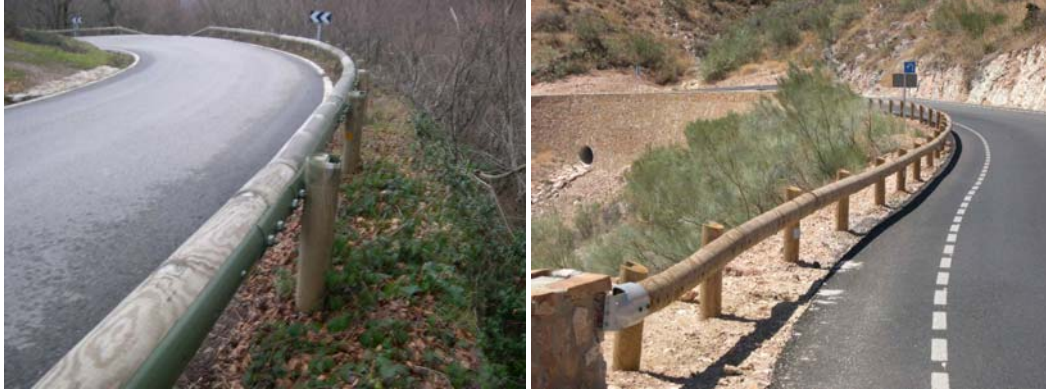
Fig. 18 and 19. Wooden safety barriers in roads. They provide a sense of the natural and rural. Although as increasingly-used standard elements, they run the risk of creating a lack of identity (Photos by I. Español).
