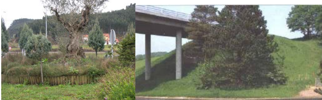
Fig. 36 and 37. Gardening and environmental recovery in road design. (Left) Olive trees and ornamental plants on a gardened roundabout. (Photo by I. Español. (Right) Environmental recovery of an embankment slope (Photo by E. Rico).
