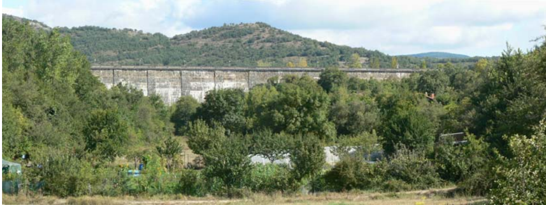
Fig. III-4. The Ullibarri-Gamboa dam seen from the A-3002 road. (Photo by I. Español)
