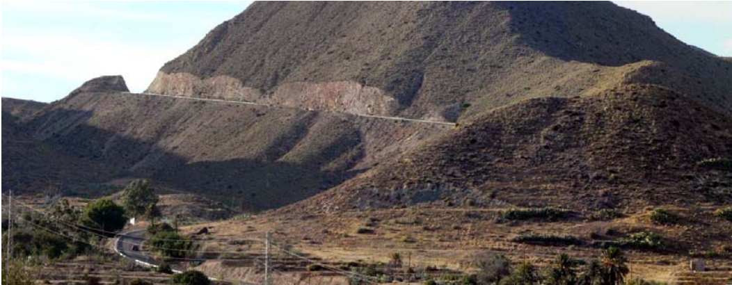
Fig. 77. Slope-cutting of roads produces a “scar effect” on landscape which can only be partially reduced by revegetation measures and rock treatments when the slope is adequate. (Photo by I. Español).
