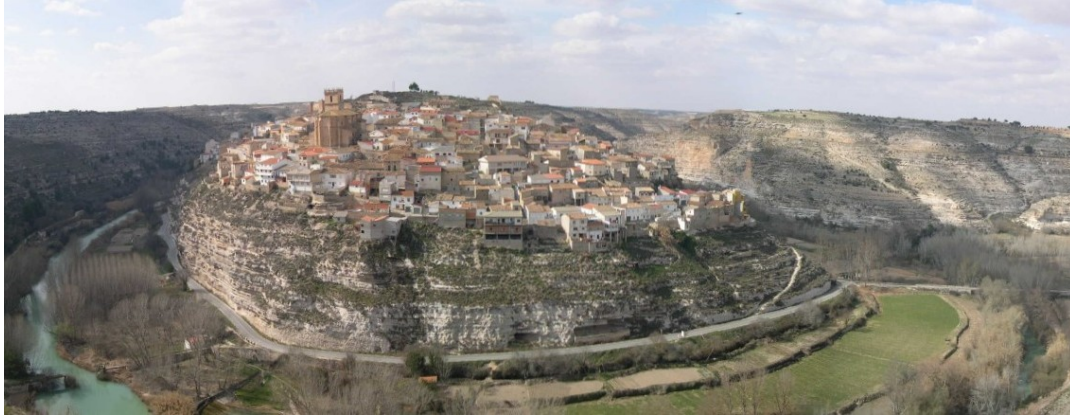
Fig. 73. The road runs at the base of the slope in this narrow valley of the River Jucar (Albacete, Spain). (Photo by I. Español) Road presence can be discreet and not imposing when its size and alignment follow basic landscape patterns.
