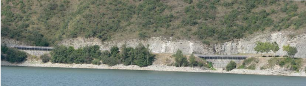
Fig. III-9. Cuttings and embankments alternate together with short bridges on the small ravines which allow slope habitats access to the reservoir shores. (Photo by I. Español)
