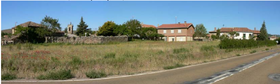
Fig. II-4. The P-220 road passing by Villavega de Aguilar where new housing stands near the parish church and cemetery (a listed monument). (Photo by I. Español)
