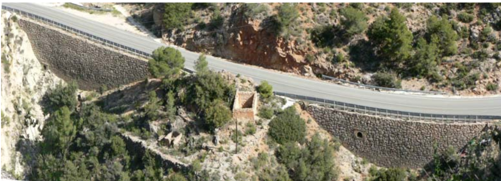
Fig. 78. Stone walls as retaining walls have a positive effect on landscape. (Photos by I. Español)
