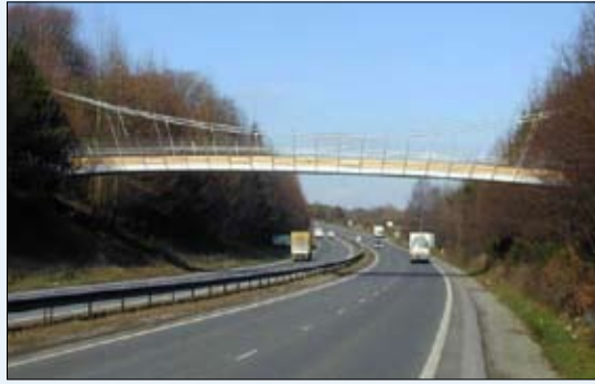
Figure 8.19 Halgavor Bridge A30. © Highways Agency
