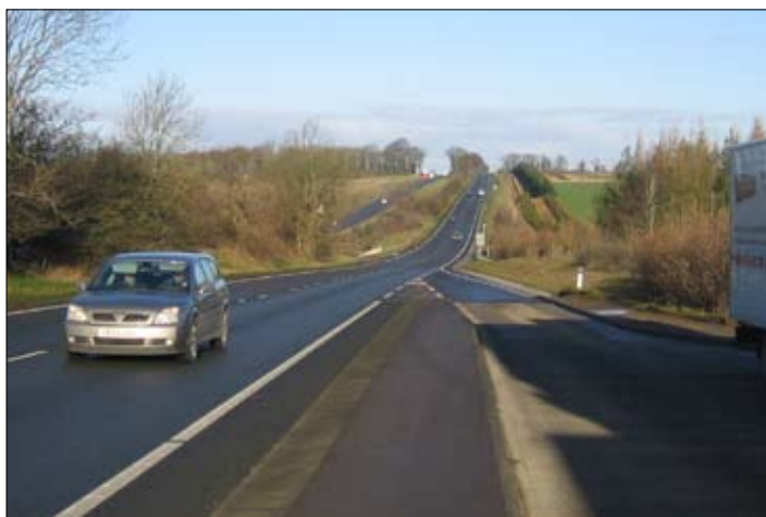
Figure 8.2 Benefit of asymmetrical widening and retention of existing boundary as central reservation in dual carriageway design – Left A417. A retained mature central reservation may help to integrate roads into their historic landscape surroundings © Halcrow Group Limited – Right - A46 Leicester © Scott Wilson Limited.
