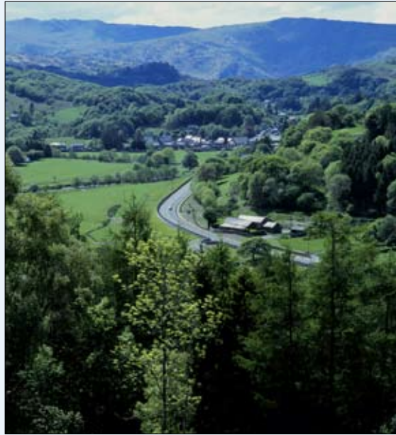
Figure 8.4 A470 trunk road between Dolwyddelan and Pont-yr-Afanc. © Colin Leftley.
