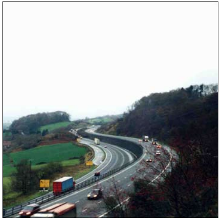
Figure 8.8 Differential vertical alignment M5 two split carriageway sections south of Bristol © Halcrow Group Limited.
