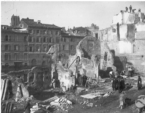
Fig. 35 _ Excavation and demolition in progress in the area of the Roman Forum, demolition of buildings in the Alexandrino district, 1932; Roma, Mediateca
