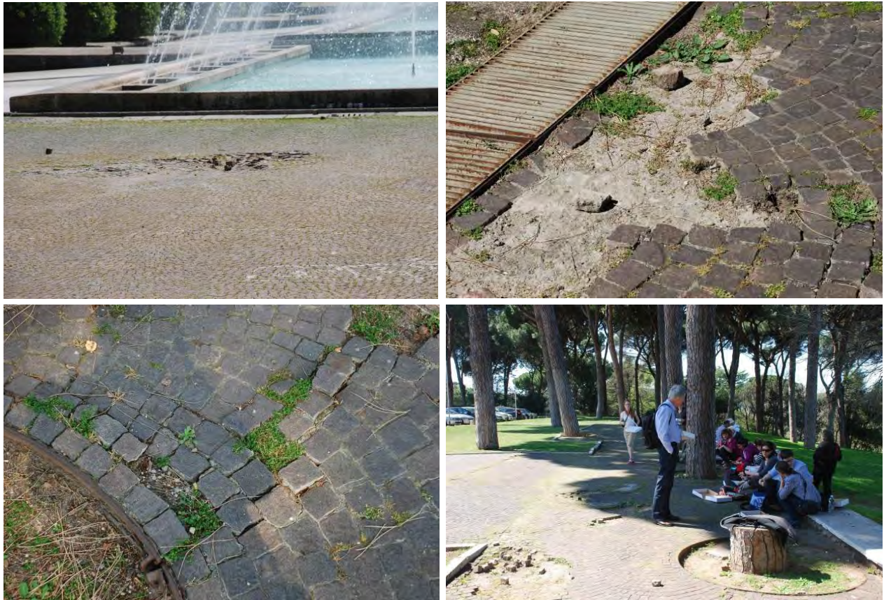
Fig. 32 (a-d) _ Technical condition of pavements in the EUR area limits the functionality and comfort for the users.
