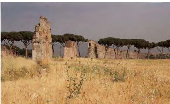
Fig. 5_ The Roman countryside, south eastern suburbs, suggestive intersection between the aqueduct Claudio and countryside
