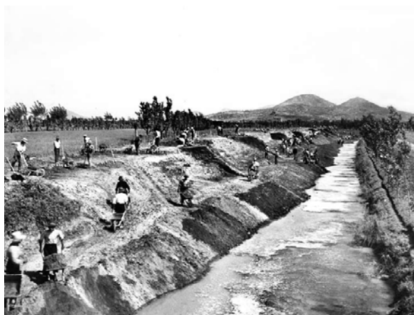
Fig. 16_ A vast project of ditch digging
