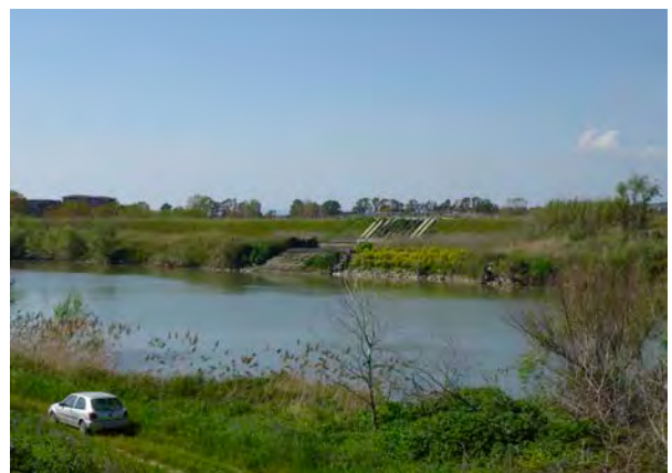
Fig. 38_ View across the river
