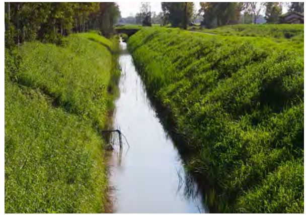
Fig. 35_ Drainage ditches are a common feature
