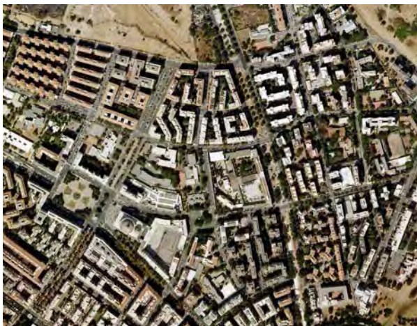
Fig. 39 _ Don Bosco district; Google Maps, aerial photo.
