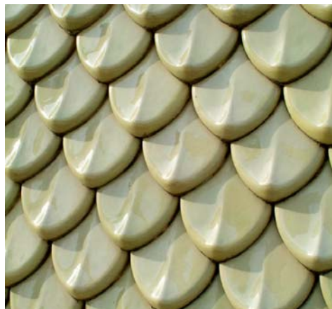
Close-up of the roof of the Casa de la Punxa (Girona, 1918) by Rafael Masó, inspired by the wheat fields just outside Girona
